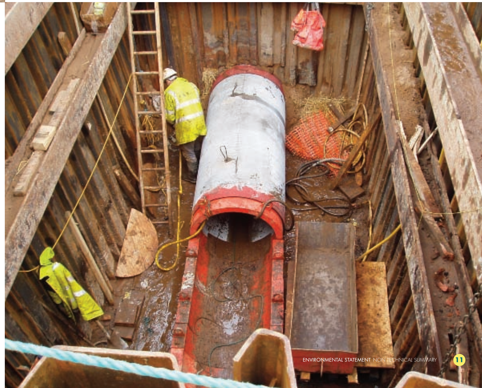
Example of tunnelling below roads
